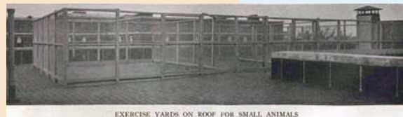
The small animal exercise yards were located on the roof at 180 Longwood Ave., 1915.
