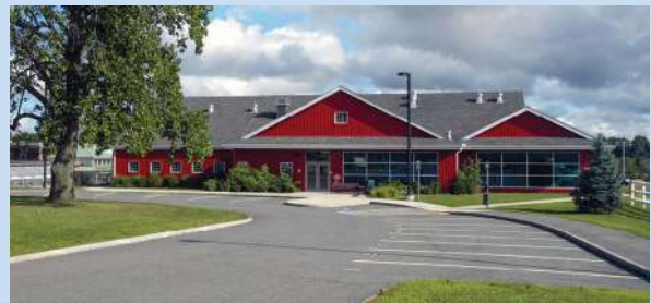
Angell at Essex on campus at Essex North Shore Agricultural and Technical School (Danvers, MA).
